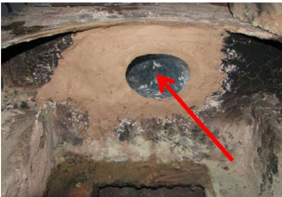
Figure 4: Pipe set into the back wall with clay
